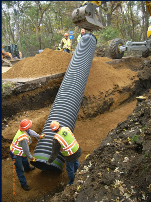
Trench New Pipe
